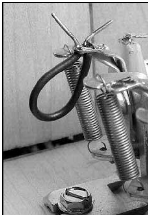
Figure 35. The cable guide ring installed, not yet trimmed.
